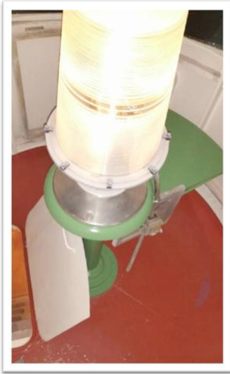
When all repairs were complete, new paint, in historically accurate colors, transformed the lantern room. The floor is now reddish-brown, the light pedestal spruce green, all interior walls – both wood and metal – are white, and the brass is clean and bright. The light shines again!
