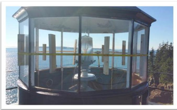
The glass panes were temporarily replaced with plexiglass panes, braced with wooden battens and wrapped with a ratchet strap.
