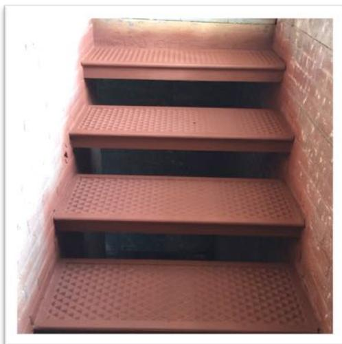
After the stairs were cleaned down to the metal, they were painted top and bottom using high quality paints in the historic reddish-brown color that was used on these stairs in the 1930s. Amburg built wooden staging inside the tower in order to reach the underside of each stair.
