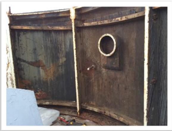
Once the wainscoting was removed, the inner face of the exterior metal wall was revealed. Rust and paint were stripped and necessary repairs were made to the metal.
