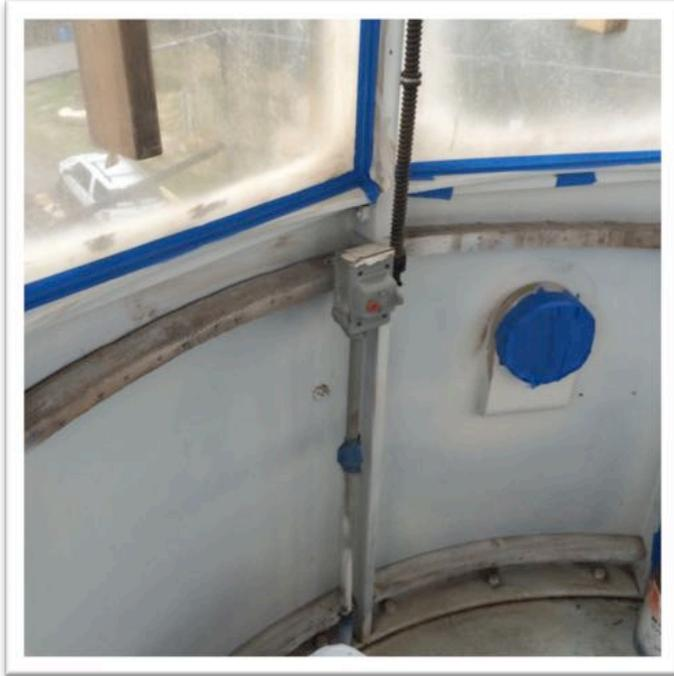
Once the interior metal wall had been stripped of rust and lead paint, Amburg made necessary repairs to the metal.
