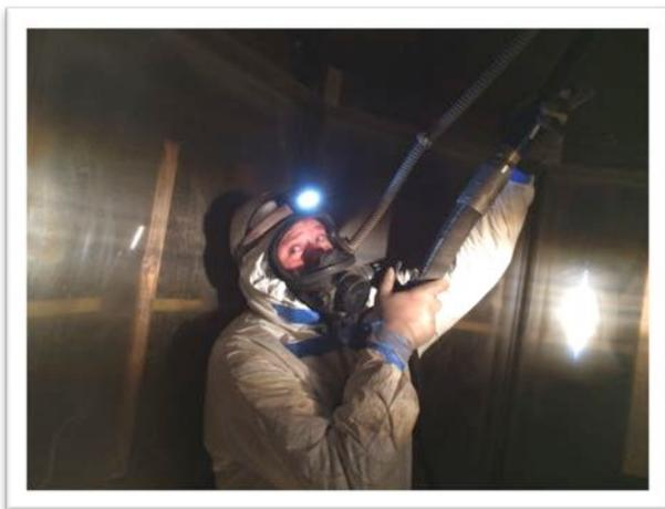
Rust and lead paint were removed from the stairs and other metal surfaces using SpongeJet equipment and a specialized blasting material. Where the stairs were set into the masonry, rust was removed up to a half inch into the masonry. Amburg was punctilious about using lead safe procedures, and disposing appropriately of all blasting debris.
