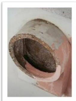
The photo on the left shows a metal vent in the cupola wall with a hole below and to the right through which daylight is visible. The photo on the right shows the same vent, after repair.
