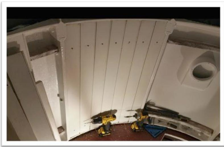
Finally, the wooden wainscoting was reinstalled. A thick caulk of beeswax was applied at the base of the wainscot to prevent future water damage. Last of all, the wood was given a final coat of paint.
