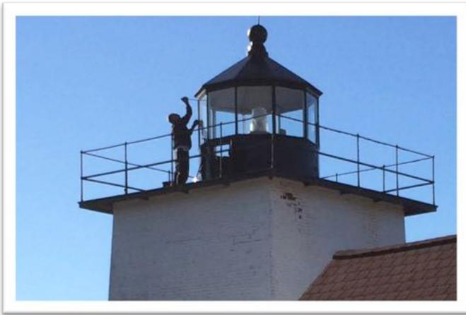
The glass window panes were removed from the cupola by Portland Glass, to allow for repair to the frames and astragals. The original glass was carefully stored.
